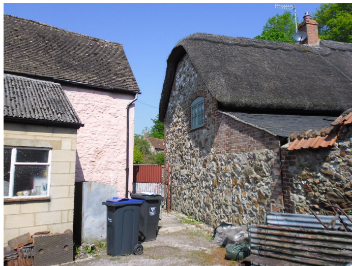
Plate 6: Rear elevation and view towards 2 Oxford Street
