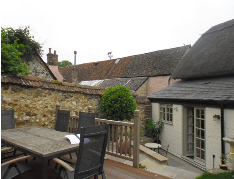
Plate 7: Rear elevation of 2 Oxford Street facing towards the application site
